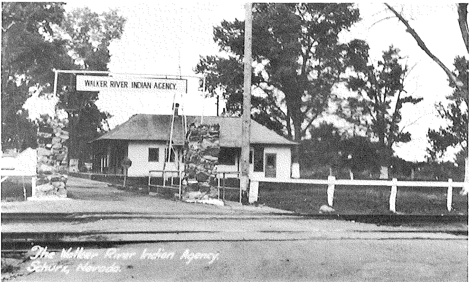
The Indian Agency building on the Walker River Reservation at Schurz. ( Nevada Historical Society )
